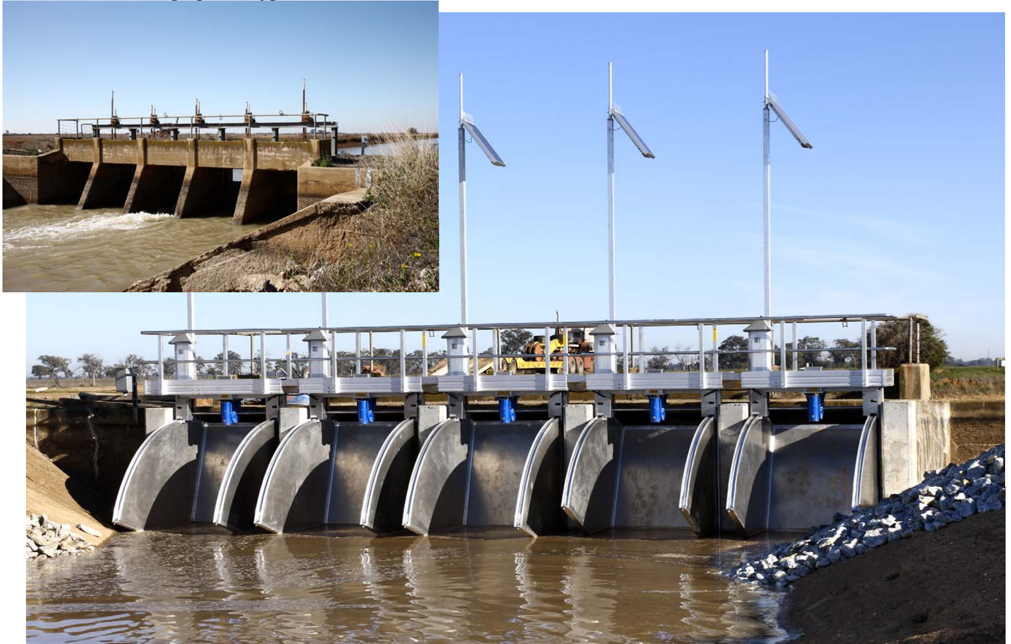
Figure 3: Before and after automation of a large channel regulator.
