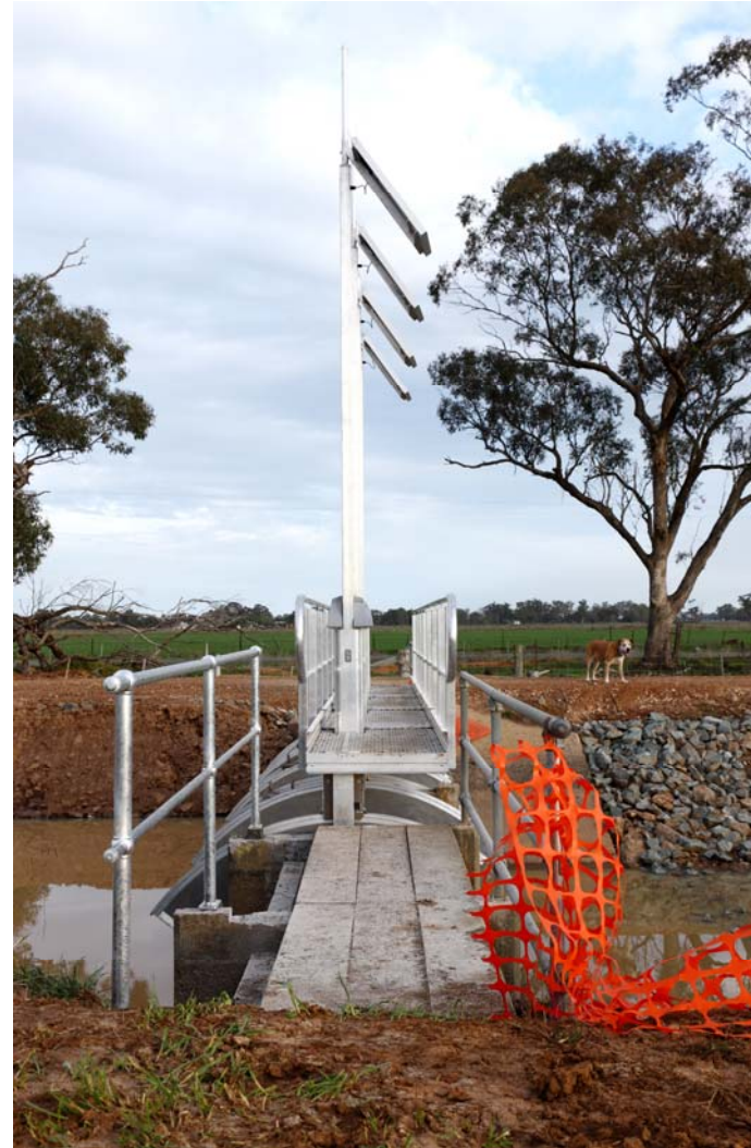
Figure 2: Gates on a channel after automation
