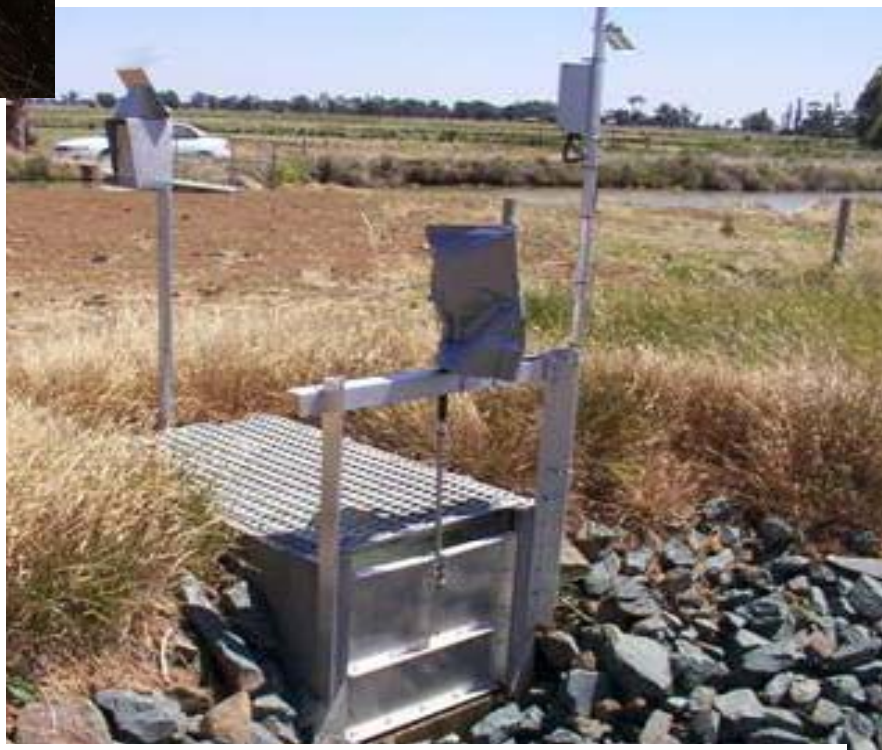
Figure 7: An installed MagFlow meter
