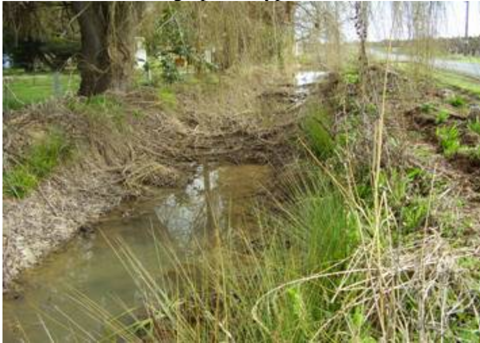
Figure 4: A channel in the Central Goulburn system before remediation works (undertaken as part of the CG1-4 Project).
